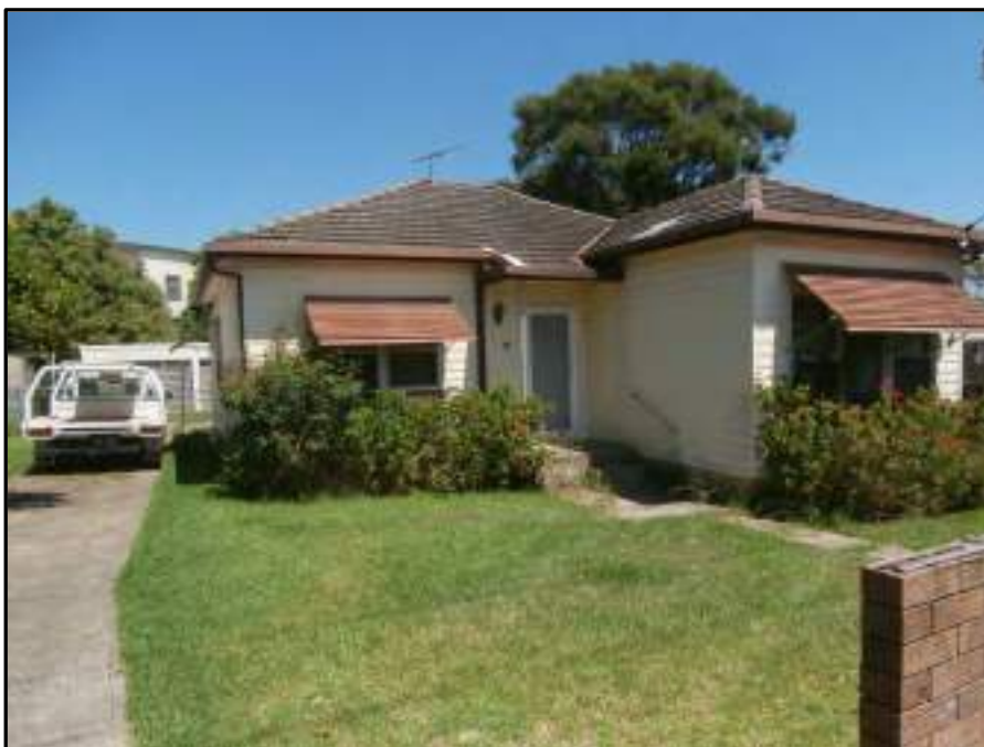
Photo 2: House on King Street to be demolished.
