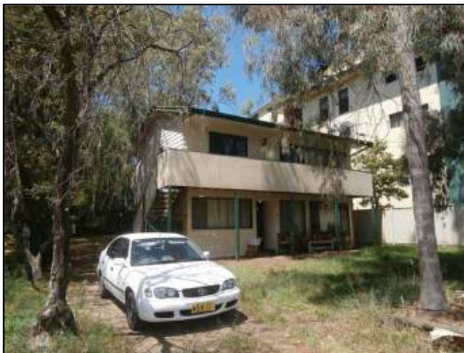
Photo 6: Dwelling on the Esplanade to be demolished.
