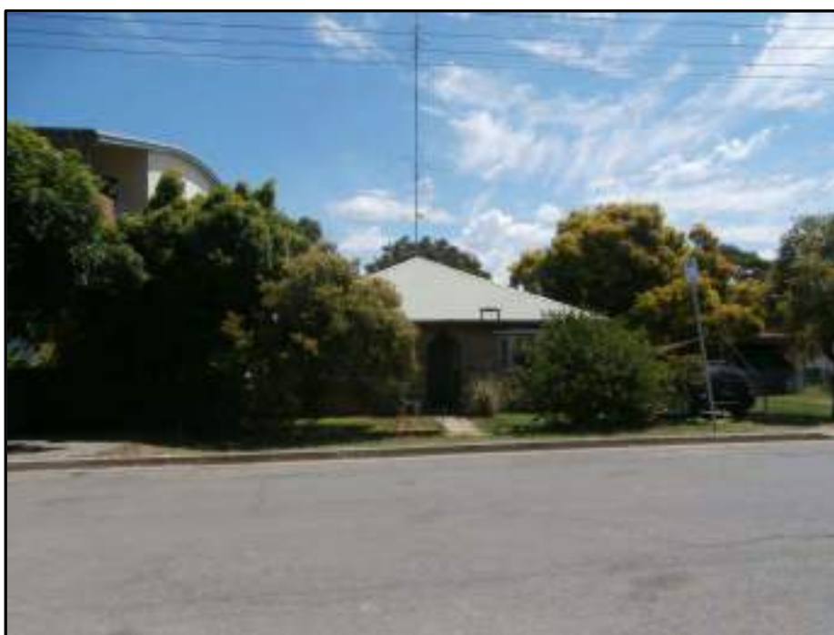
Photo 9: Dwelling on Howard Street to be demolished.
